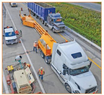
Highly-mobile barrier systems deflect very little when hit by an errant vehicle (Source: QMB Barrier).
