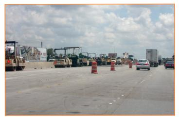
Some work zones include a large distance separating the traffic space and work space (Source: TTI).
