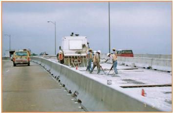
Some work zones include concrete barriers to separate the traffic space and the work space (Source: TTI).
