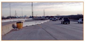
Barrier ends in work zones must be protected by flaring them and/or providing crash cushions (Source: TTI).
